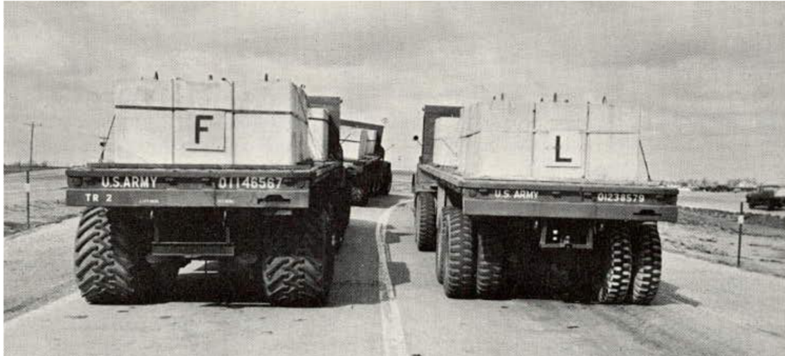
Figure 1.5: AASHO Road Test. Example of experiment comparing the effects of a low pressure-low silhouette tires (left) and conventional tires (right). [BOA 62]
