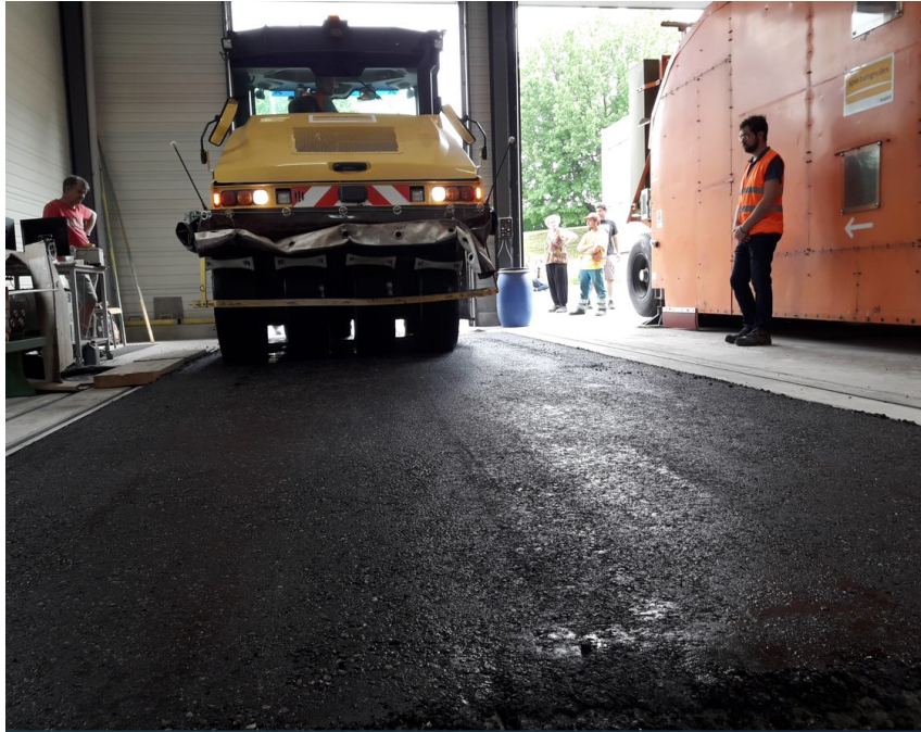
Figure 7.25: Building the pavement structure for the experimental investigations in GC2D.
