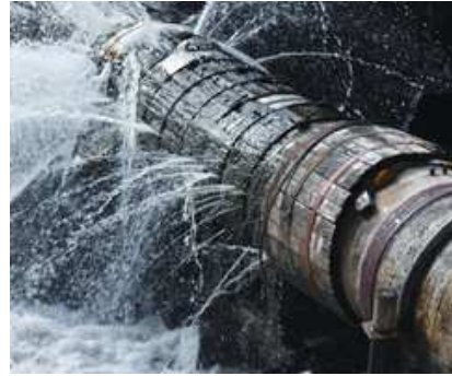
(b) Fracture of water pipe.
