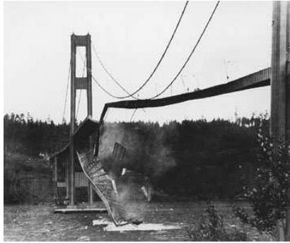
(a) Collapse of Tacoma Narrows Bridge (1940).
