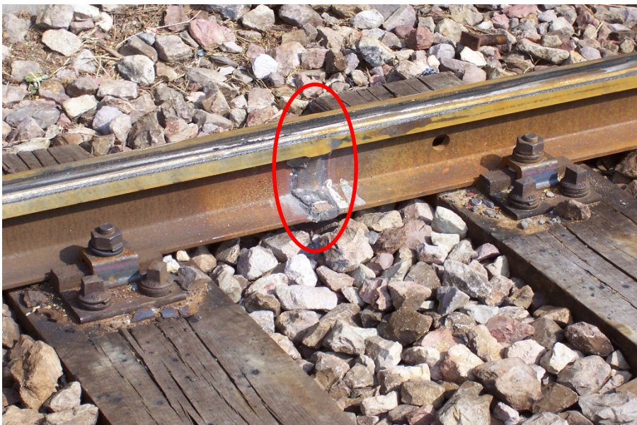
Figure 4.7 Welded rail joint[69]
