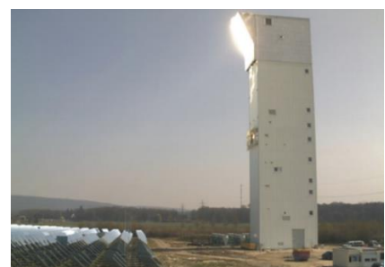
Fig. 0.8 – Jülich solar tower [11]
